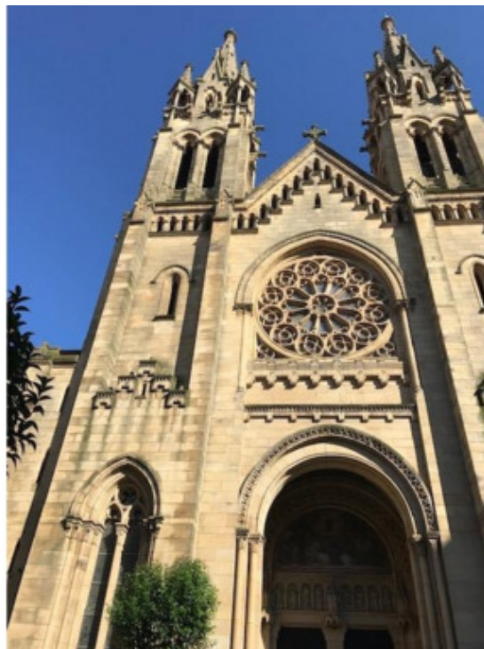
Fig. 225. Church of St. Francis of Assisi.
