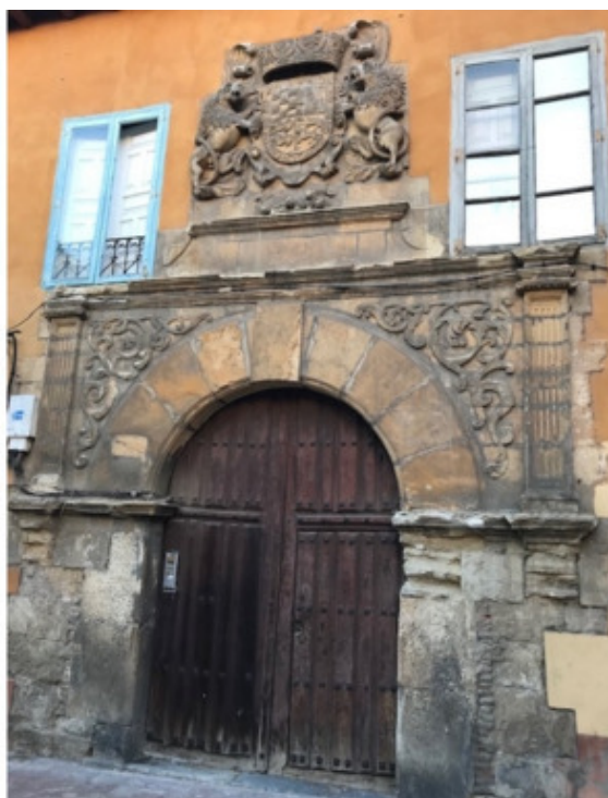
Fig. 193. The old entrance to the building.
